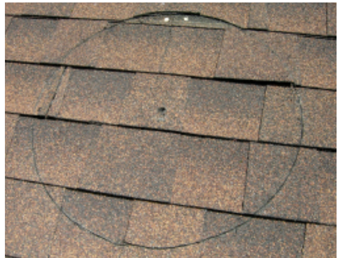
Diameter of hole to be cut marked on shingles.
