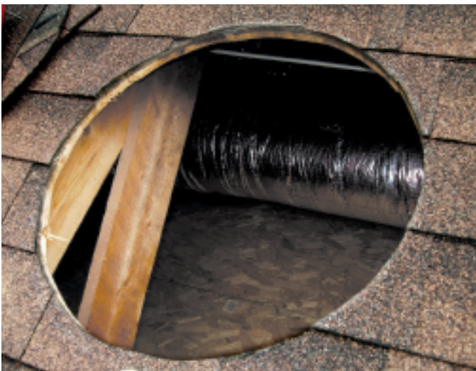
Hole cut with reciprocating saw.
