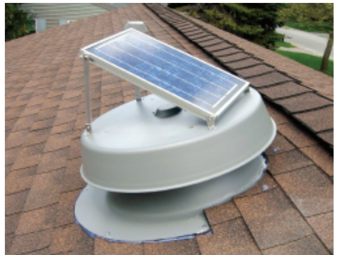
Unit installed , seams caulked and solar panel angle adjusted.
